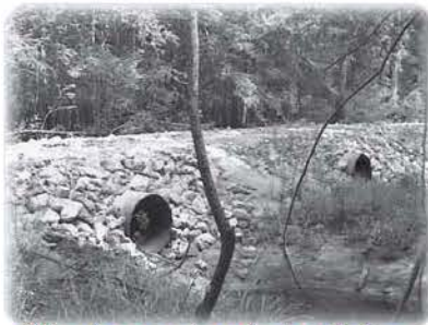
Culverts are an important part of reducing sediment from road systems.
