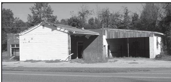
Left: Campbell's Service Center had fallen in disrepair.
