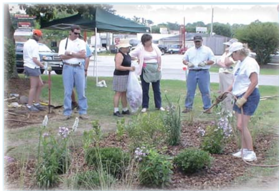
Installation of a rain garden in Surfside Beach.
