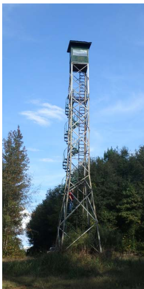
Anderson/Greenville/Oconee/Pickens Project Forester Trey Cox sent in this photo of the tallest deer stand he's ever seen. It was constructed using a high-tension line base for powerlines by Ted Wheeler of Pendleton. He erected it section by section with the help of a friend who owns a crane.
