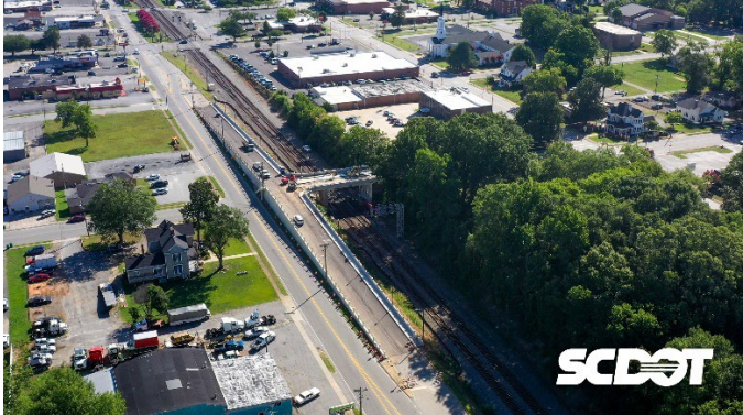
Image 1 Gaffney T-Bridge under construction
