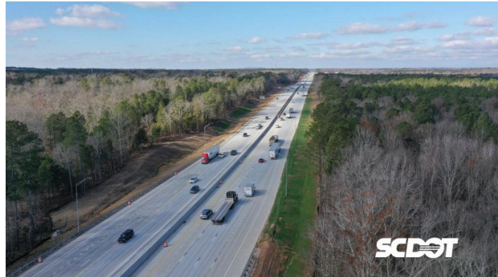
Image 2 Midlands Connection Project on I-26
