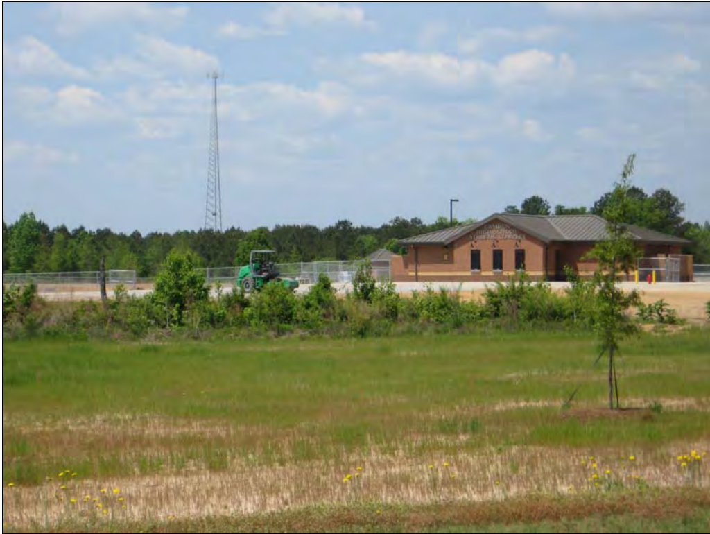
Photo 7: View of Camden High School Athletic Field Complex, looking east.
