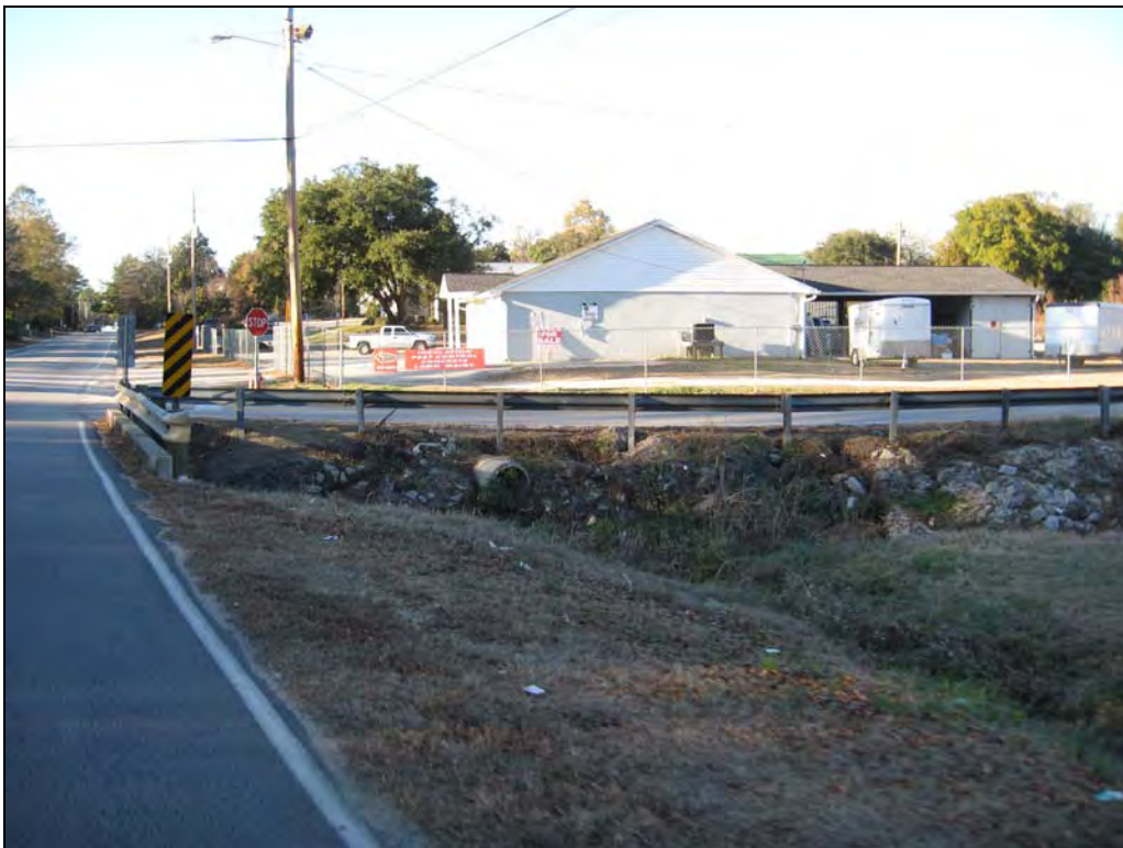
Photo 6: View of Chestnut Ferry Road crossing Bolton Branch Creek, looking west.
