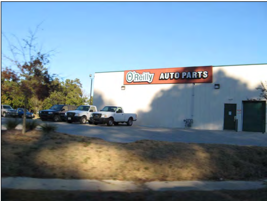
Photo 10: View of commercial development, looking northeast.
