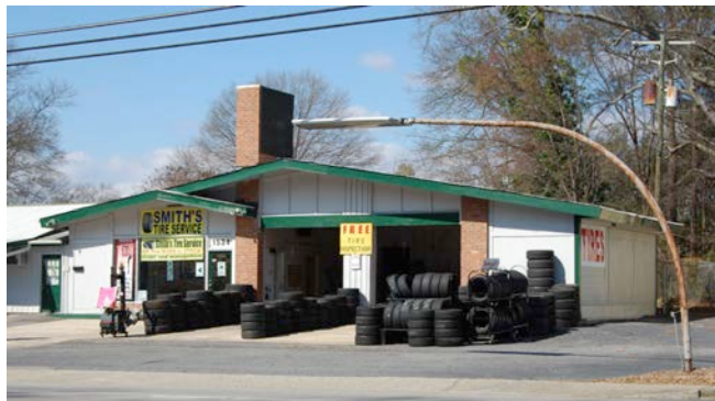
Renovated gas station with low-sloped roof, large "chimney" stack and glazed gable are still evident. Note the Modern site lighting fixture. West Columbia, SC.
