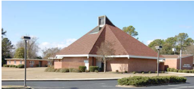
The campus of Our Savior Lutheran Church includes the Education Building (1966) background left, and the Sanctuary (1971-74), West Columbia, SC.
