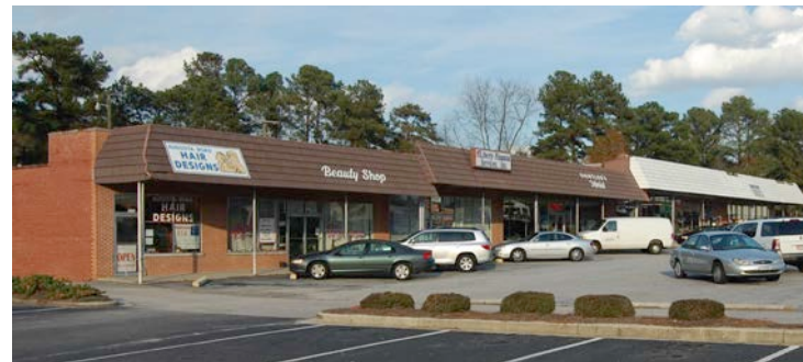
Lowntown Shopping Center, West Columbia, SC. The Mansard-type roof over the sidewalk was added much later. The original corrugated metal awning is visible beneath.
