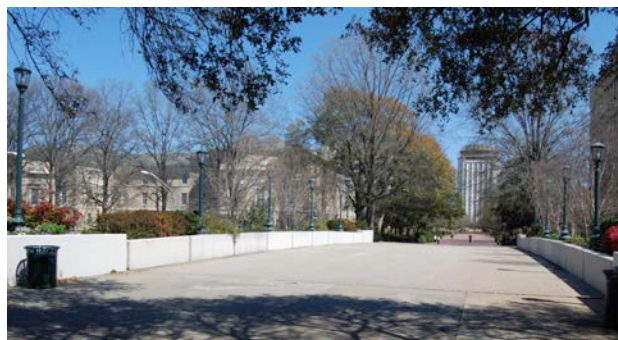
USC Pickens St. Pedestrian Bridge (1973), Columbia, SC.
