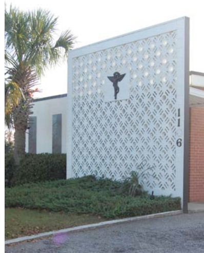
Decorative masonry screens, like the one at 1106 12 th St., West Columbia, SC were common in 1960s architecture.
