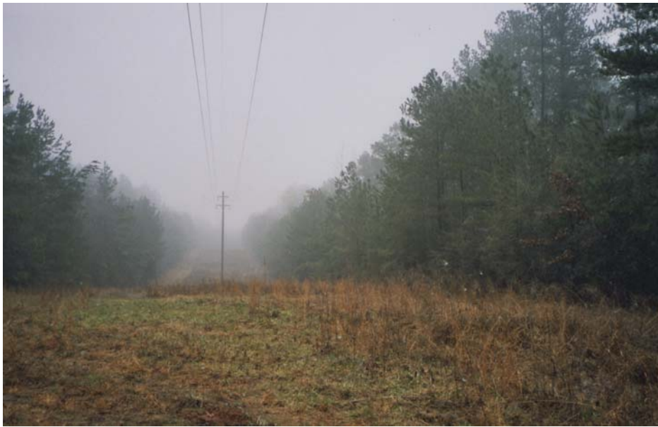
Figure 4. View of the existing transmission line and the project area.
