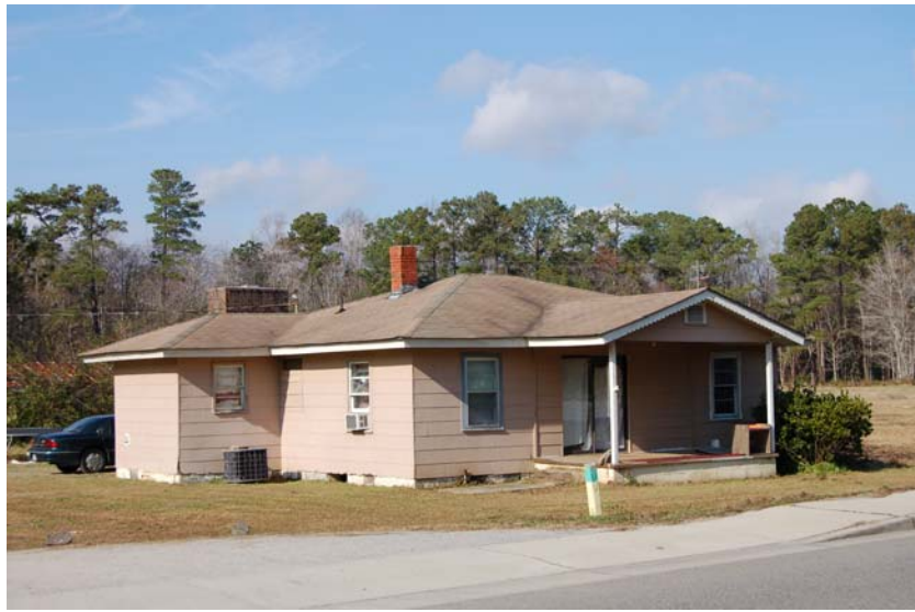
Figure 12. View of Structure 060-0064.
