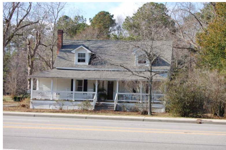
Figure 13. View of Structure 060-0503.
