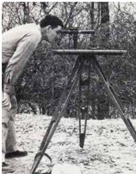
Young Nick Zeigler peers through an engineer’s level while on survey with Philip Phillips in Mississippi in 1949 (Williams 1970:30).
