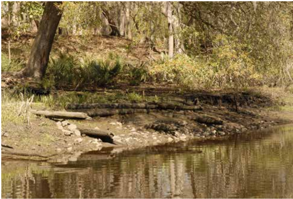
Fig. 3: Remains of the colonial cribbed dock at Fort Dorchester. (Photo by Drew Ruddy)
