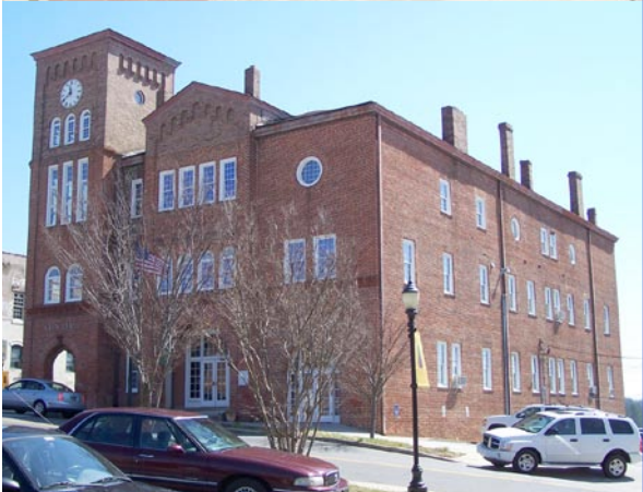
A S.C. Preserve America Initiative grant is funding a preservation plan for the historic Chester City Hall.
