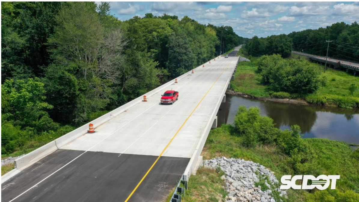
A new bridge is open to traffic on US 301 southbound over the South Edisto River in Orangeburg County.
