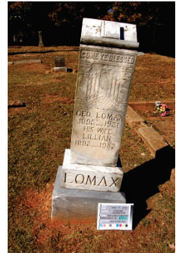
Example of a Priority 1 repair, this stone could easily be toppled, injuring visitors to the cemetery.
