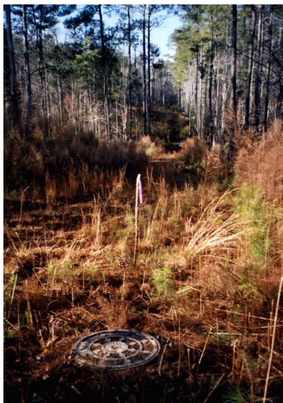
Figure 14. Existing sewer line near the Stonington Subdivision.
