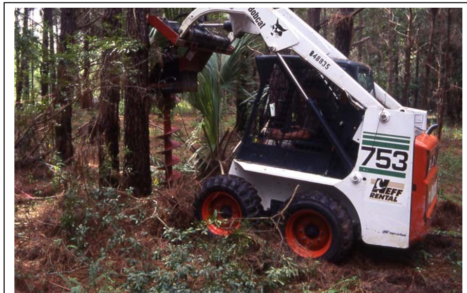
Figure 5. Use of Bobcat and 12-inch auger to conduct close interval tests.
