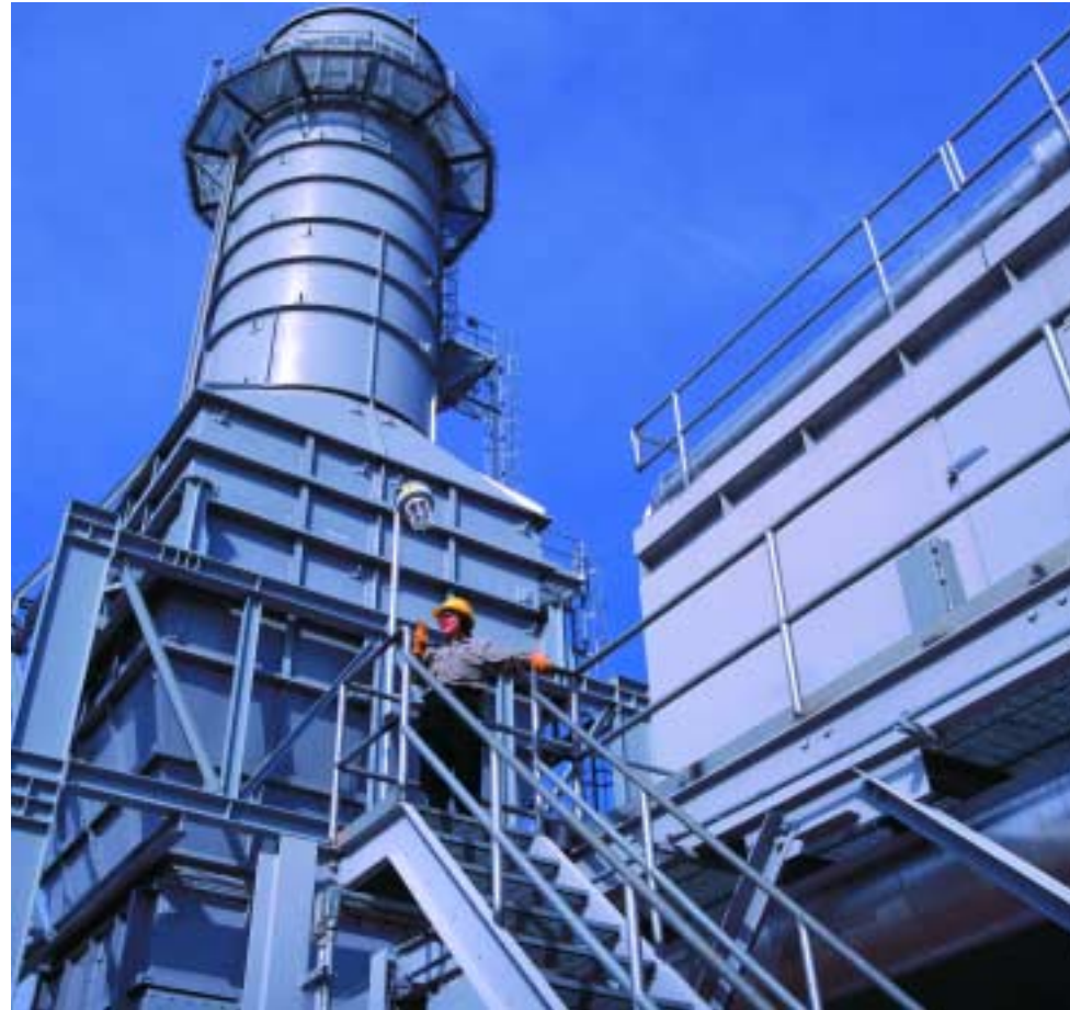
Right: A natural gas-fueled combustion-turbine generating unit starts up at Rainey Station in Anderson County.
