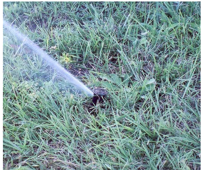
Figure 4. A gear-drive or rotor sprinkler in operation. (Photo credit: Bryan Smith)
