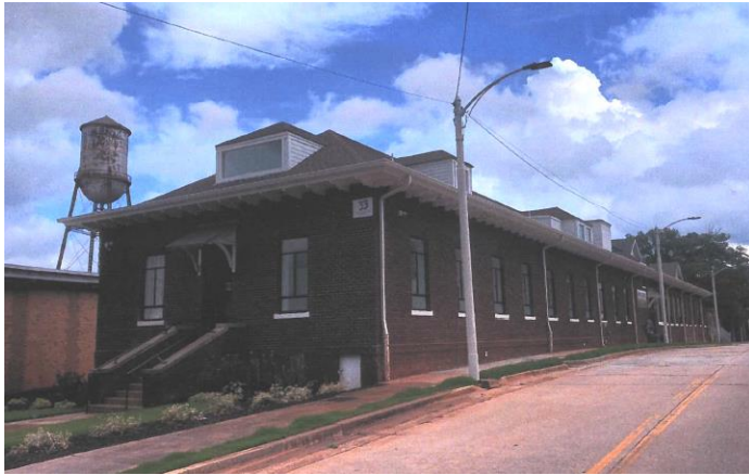
Dunean Mill Office building after rehabilitation. Image courtesy of Kyle Campbell.
