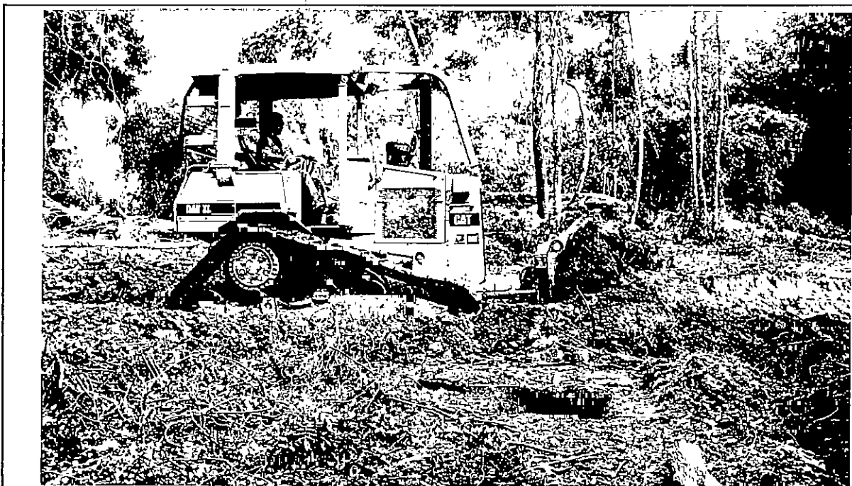
Figure 18. Bulldozer stripping off an area south of the posited earthwork, view to the north.
