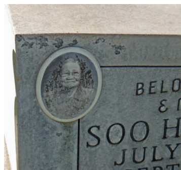
Dissolved minerals are coating this stone, obscuring the porcelain photograph.
