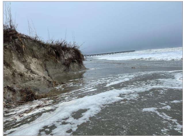
Erosion at the Isle of Palm. Courtesy of J. Sovine.
