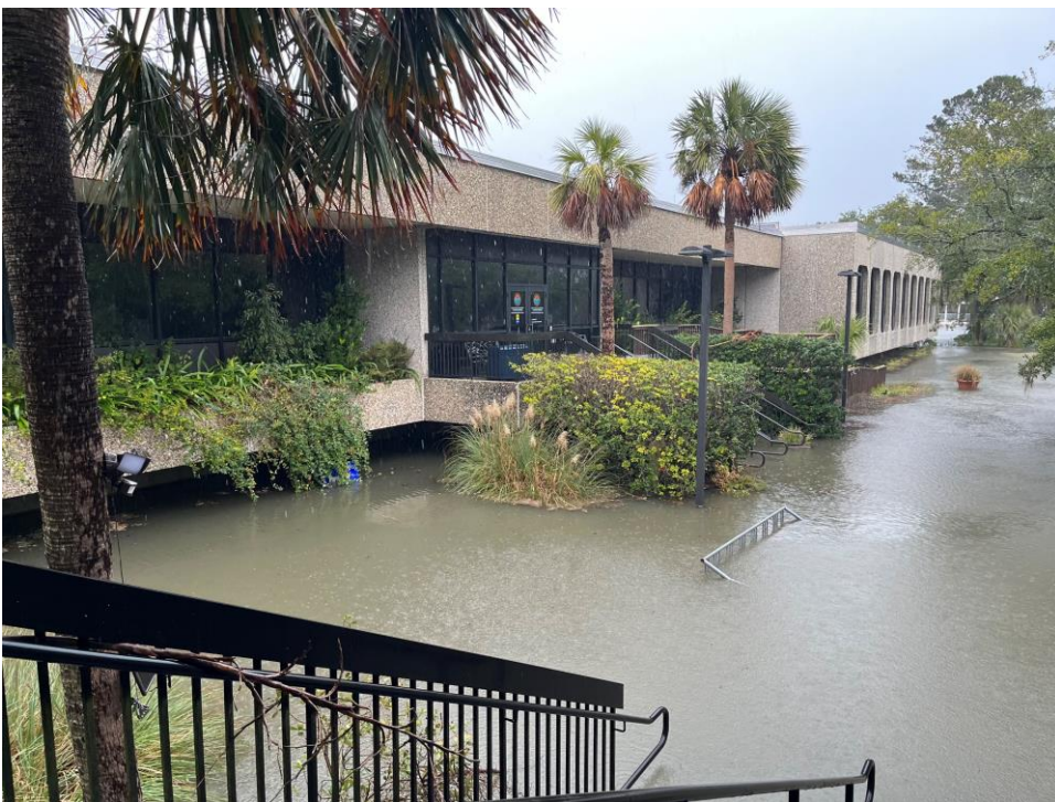
Flooding at the SCDNR Marine Resources Division Headquarters facility at Fort Johnson.
