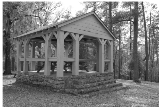
Coquina was used for shelter #5's foundation and steps. This shelter was started by Company 421 and finished by Company 4475.
