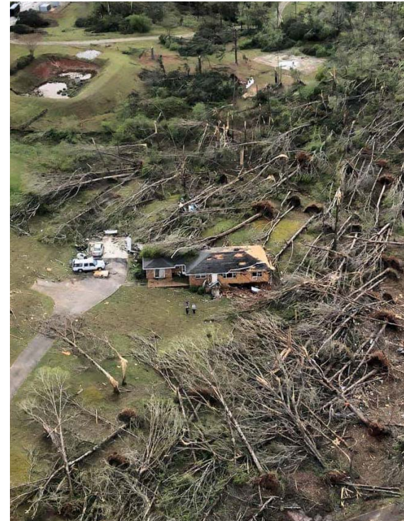
EF-3 Tornado damage in Seneca.
