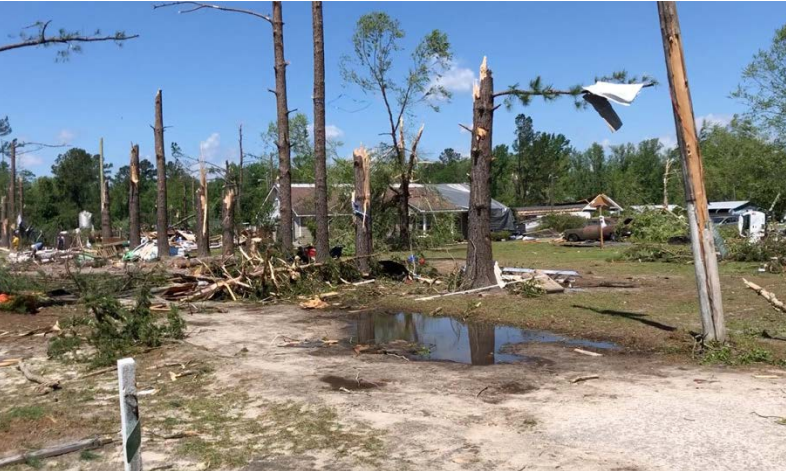
EF-4 Tornado damage in Hampton County.
