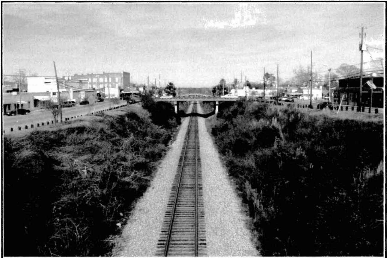
Figure 2 - Present View of St. Matthews Railroad Cut
