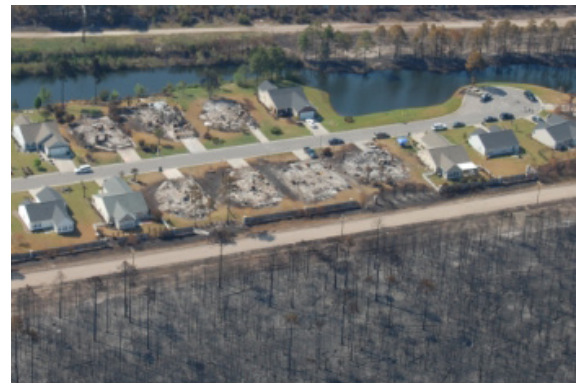
In 2009, 76 homes were destroyed and 97 damaged during the Highway 31 Fire.
