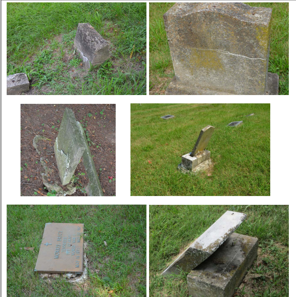
Figure 15. Examples of stone damage that requires conservation treatments. Upper left photo shows a broken die on base. Upper right is a cracked die on base. Middle left is a spalling limestone. To further complicate its preservation, the stone has been set in Portland cement, which must be carefully removed. Middle right is a tab in socket that is loose and requires resetting with a high lime mortar. Lower left is a bronze marker that has become detached from its base. Lower right is a die on base with ferrous pins. Repair of this stone will require drilling out the ferrous pins and replacing them with non-corrosive stainless steel or fiberglass.
