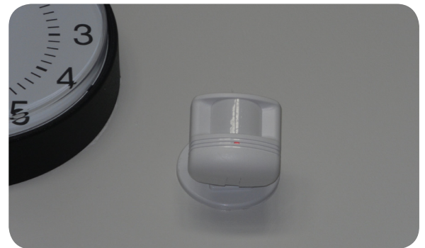
Programmable thermostats keep temperatures consistent, reducing energy usage (top) and motion sensors installed in district classrooms help keep costs down while rooms are unoccupied (bottom).
