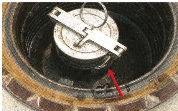
Photograph 2: Slip-on spill containment basin with a cracked collar
