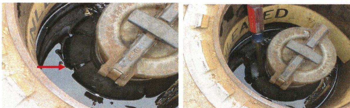
Photograph 2: Slip-on spill containment basin with a cracked collar
