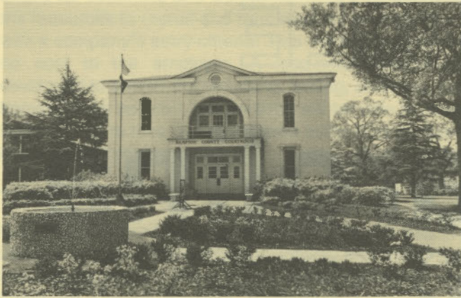
Hampton County Courthouse
