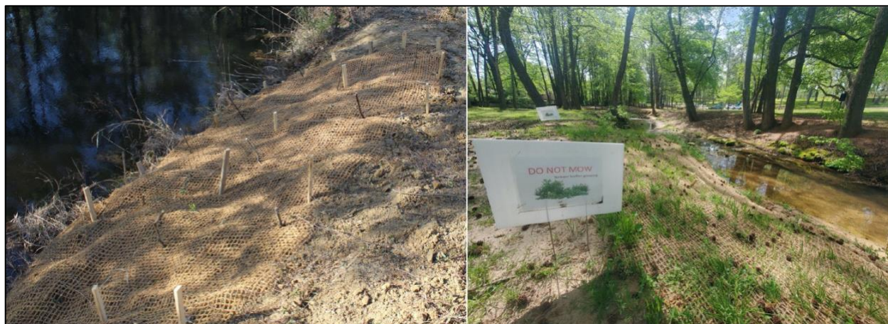
Figure 21. Streambank stabilization to minimize bank erosion and nutrient losses (Image credit: Clemson Extension, Stream Bank Repair Manual for South Carolina ).
