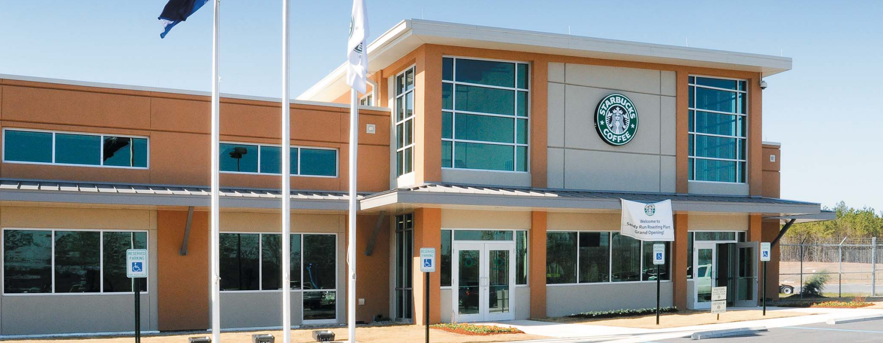
STARBUCKS' NEW ROASTER IN CALHOUN COUNTY, S.C. WAS CONSTRUCTED WITH A FOCUS ON ENVIRONMENTALLY-CONSCIOUS TECHNIQUES AND MATERIALS.
