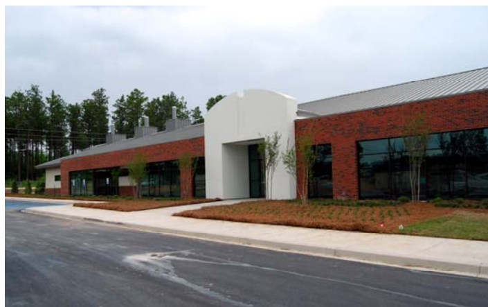
New Laboratory and Consumer Services Facility Figure 7.1
