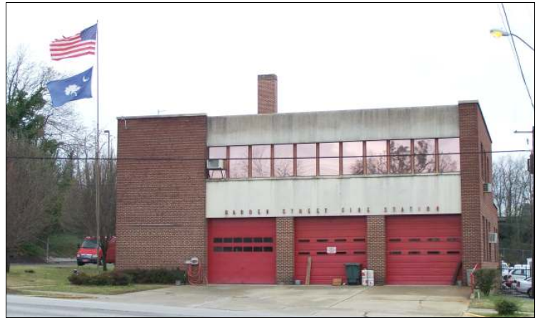
Harden Street Substation, built in 1953, employed the city Fire Department's first African American firemen. It represents a duplicative space from institutional segregation.
