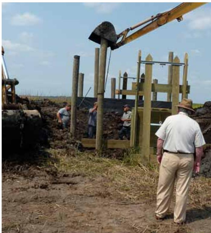
Figure 2. Installation of a new rice trunk at Long Brow Plantation.
