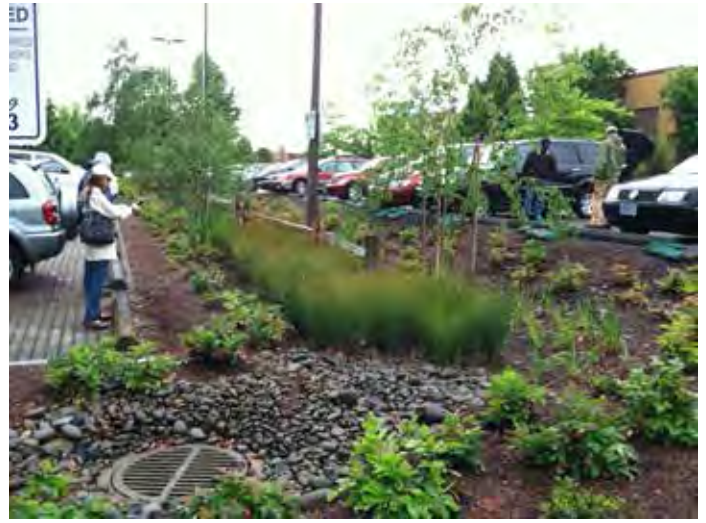
Fig. 2 Bioswale in a parking lot in Portland, OR.
