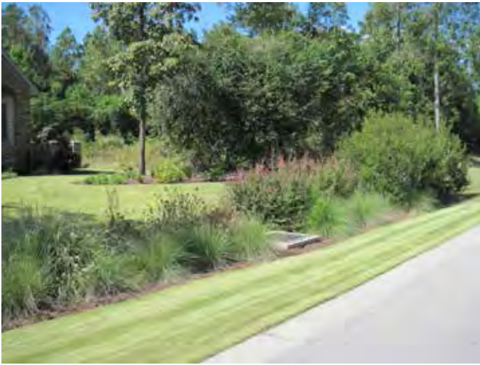
Fig. 1 Vegetated bioswale in front of a home in The Cove subdivision in Sumter, SC.
