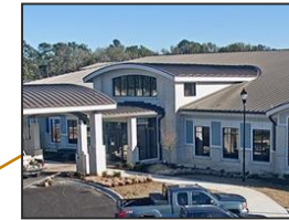
Veteran Village Skilled nursing care facility in Florence for SC veterans. Expected to open in 2021..
