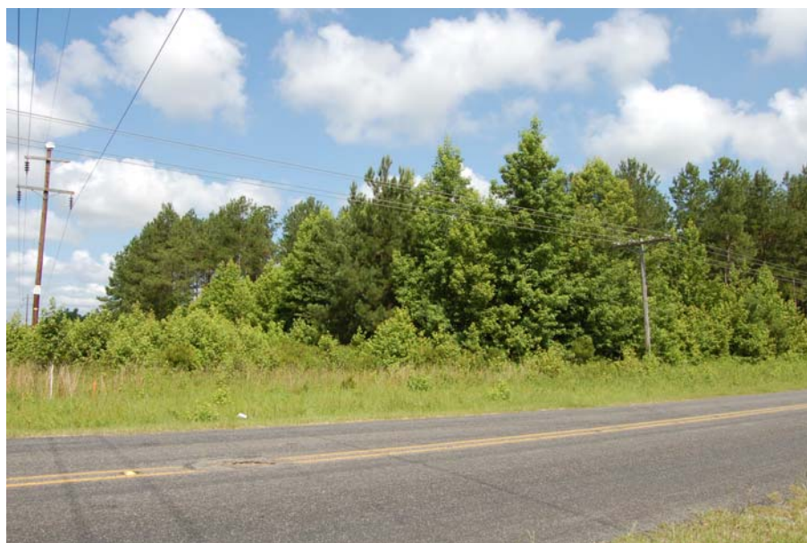
Figure 8. View of substation with existing transmission line to the south.
