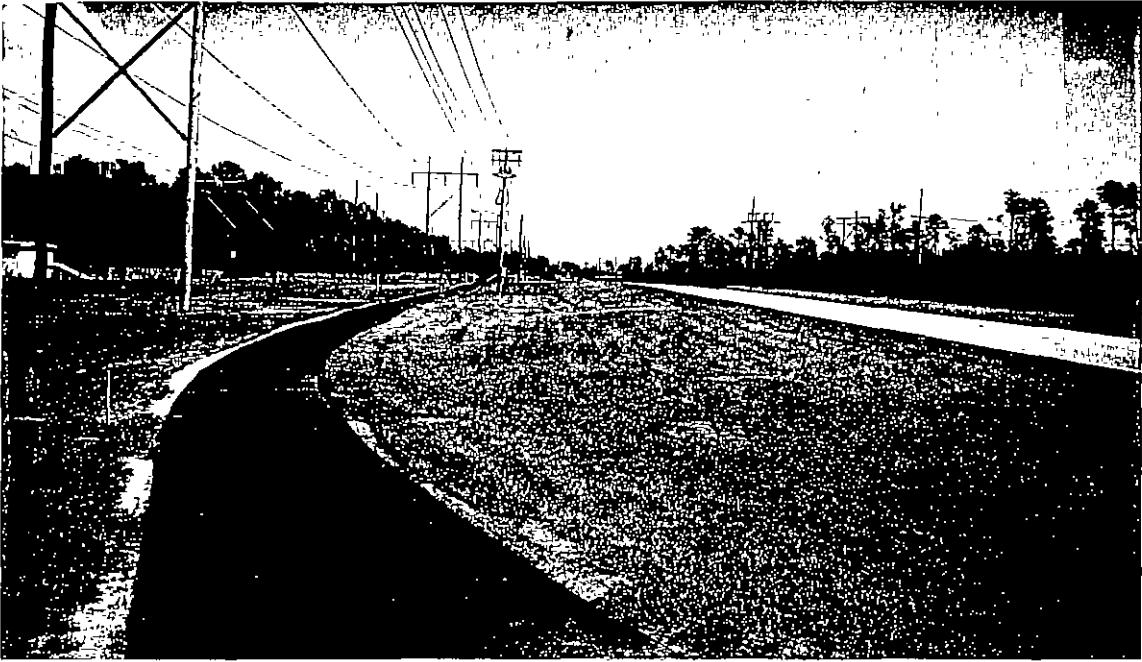
Figure 3. Survey corridor along north side of Red Bank Road, just east of the sewer facility, looking east.
