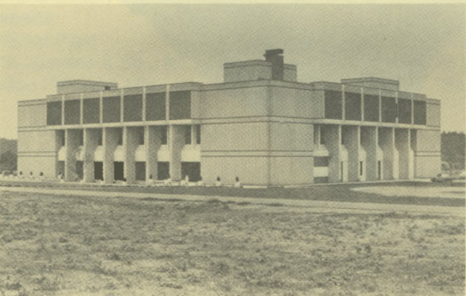
Greenville Technical College Administration Building
