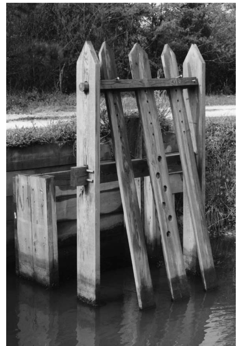
Ricfield trunks, similar in design to those used by rice planters two hundred years ago, now control water levels in impoundments managed for waterfowl and other wildlife species.
