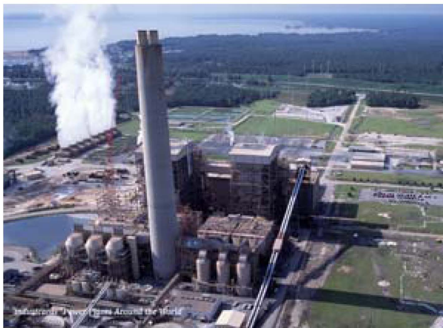
Santee Cooper's Cross power plant, located in Berkeley County
