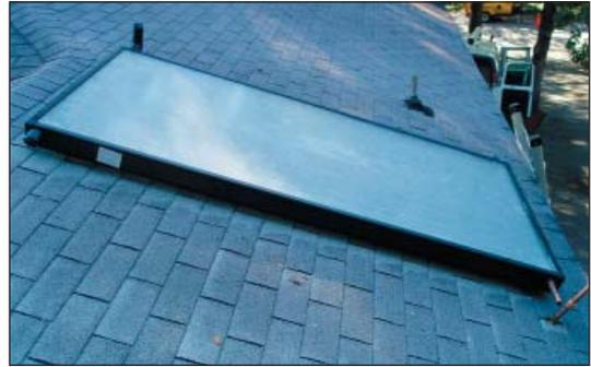
Viji and Bala Sashikant of Columbia installed a solar water heating system on their home using a 4 x 8 solar thermal collector roof-mounted panel. A digital controller monitors and displays the real-time operating temperature.
