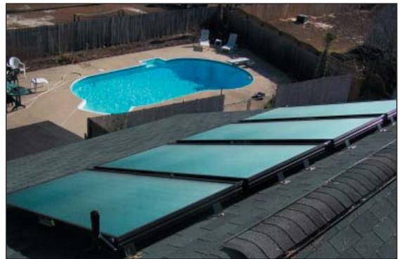
Brett Parks of Lexington has a heliopak dual solar water heater and pool heating system. The setup can get over 140,000 BTUs per day when it's operating at peak.
