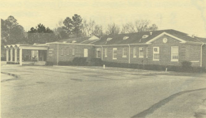
Allendale County Hospital
