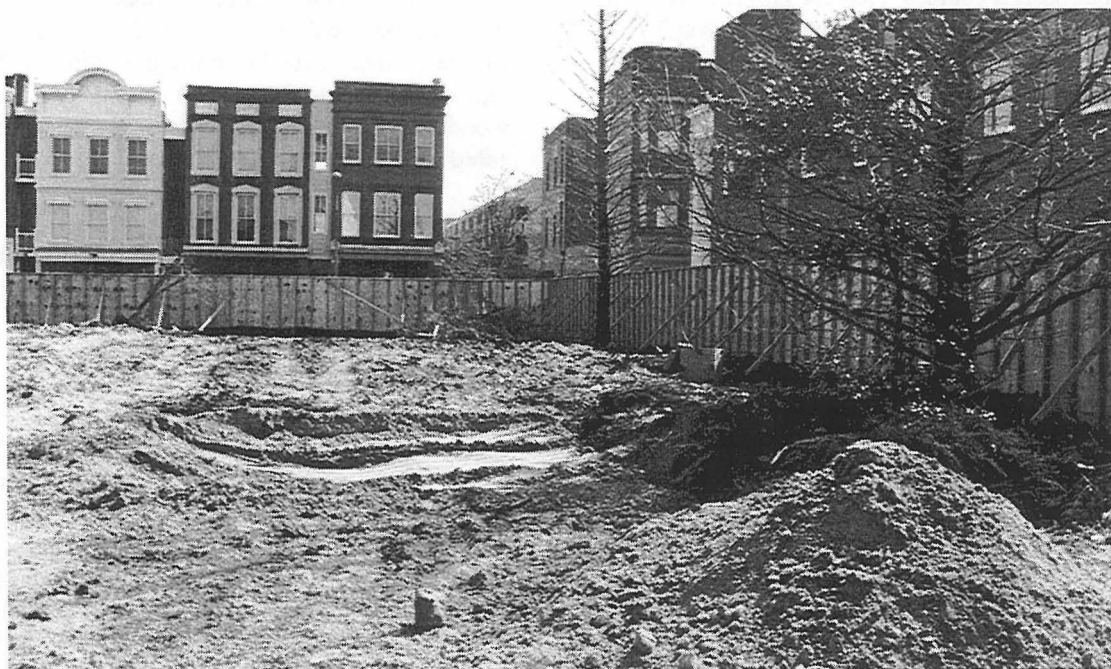
Figure 68. Area of Unit 5 with the yellow sand fill removed, prior to unit excavation. View is to the east (toward King Street in the background).
