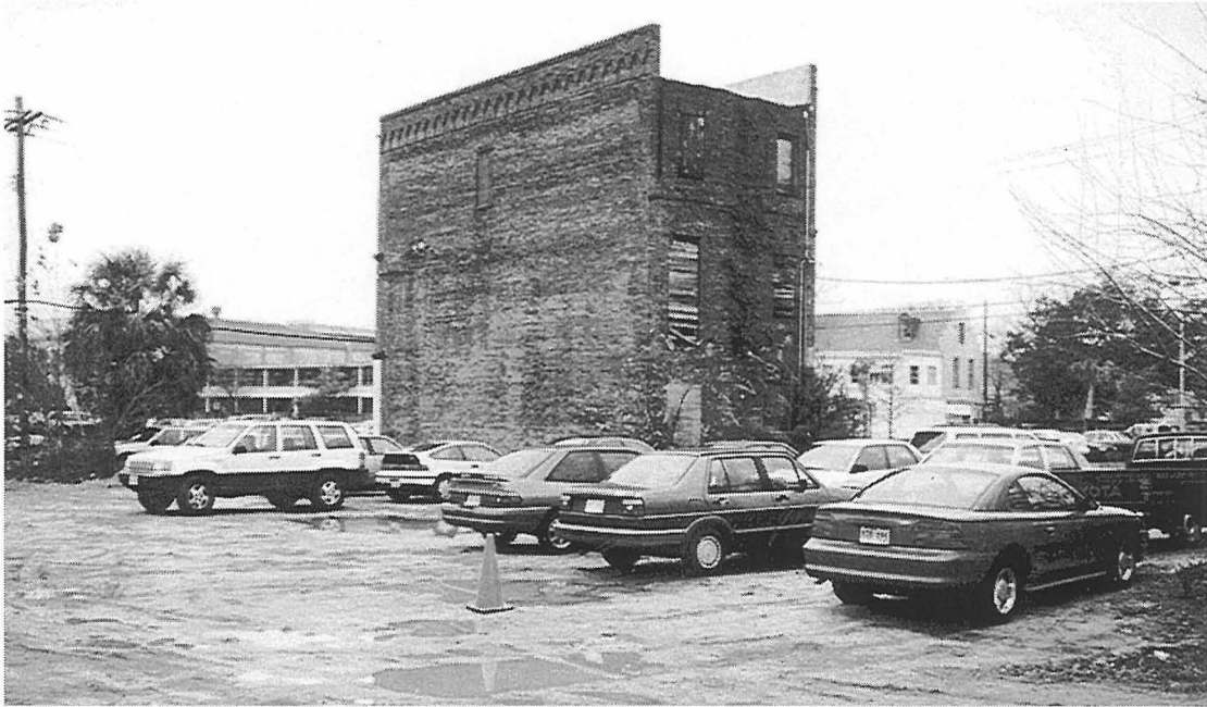
Figure 39. Western half of the project block, view toward the northwest showing the standing structure on the corner of Archdale and Market streets.
